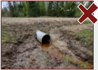
Erosion around a culvert is contributing sediment to the watercourse.
