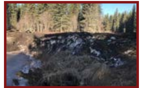
A snow fill that was not removed before the spring thaw.
