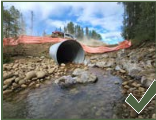
An embedded culvert outlet that has been appropriately armored with large rocks to prevent erosion.
