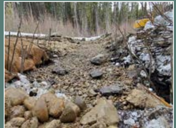
Installation of a ford surface shown while the watercourse is still frozen. Banks have been staked to promote spring revegetation. An erosion net protects the bank during construction.
