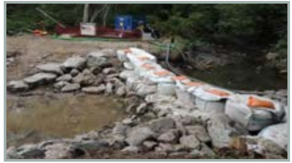
An example of a well-constructed dam across a watercourse.
