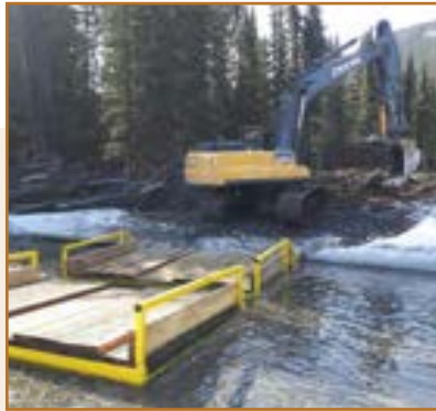
Left: A rocky and shallow section of a watercourse without steep banks that was chosen as a site to ford. Right: Portable modular bridge sections used to ford during a bridge construction project.
