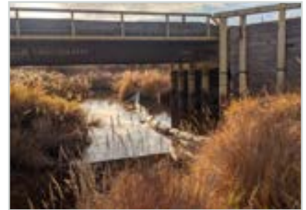
A floating sediment curtain installed around a bridge abutment.
