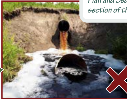
A culvert (not embedded) that was not adequately protected at the outlet. High flows have extensively eroded the crossing, causing severe issues.
