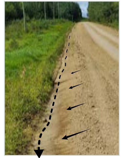
A false ditch at the side of a gravel road. Rainwater from the road flows along the edge instead of into the vegetated ditch.
