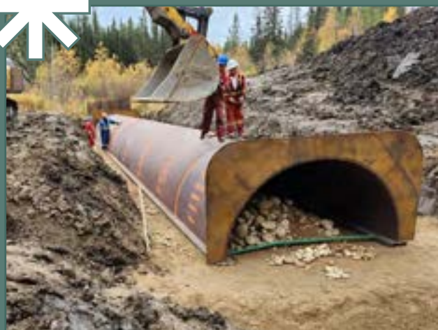
Installation of an arch showing steel footers that run the full length of the arch walls. The footers are supported by a well-compacted base.
