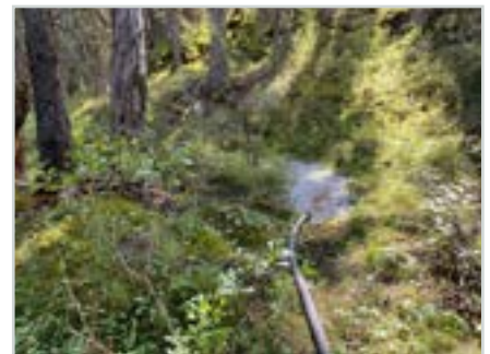
Seepage water being pumped into a vegetated area away from the watercourse.
